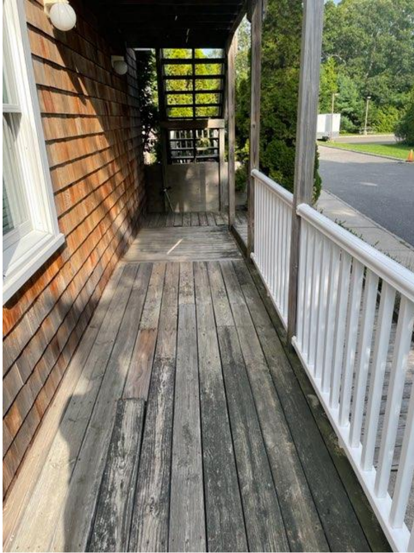
Wheel chair ramp to building
